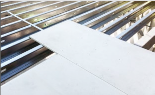
Subfloor over steel joists
