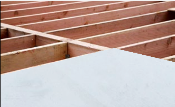
Subfloor over wood joists
